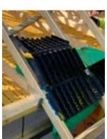
**Step 4:** Fix rafter tray into finished position with nails or staples into rafter.
