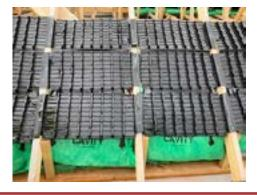
**Step 3:** Fold out rafter tray to finished position this ensures rafter tray is not compromised by loft insulation to be installed later, position large piece of insulation between bottom chord of roof trusses.
