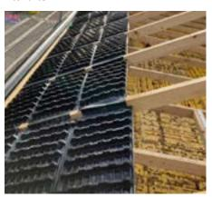
Step 5 (if required): Product can be installed in truss bays at less than 600mm centres by cutting trays and detaching insulation bag. Simply cut rafter tray with knife to fit any narrow truss bays or valley areas, and detached bag of insulation can be installed below the tray the tray to ensure no cold bridge. This does not com-promise the ventilation integrity as a typical roof has been designed with more than the required 10000mm2 per lm.
